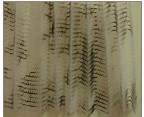
Burnt polymer pleat support mesh from arcing
